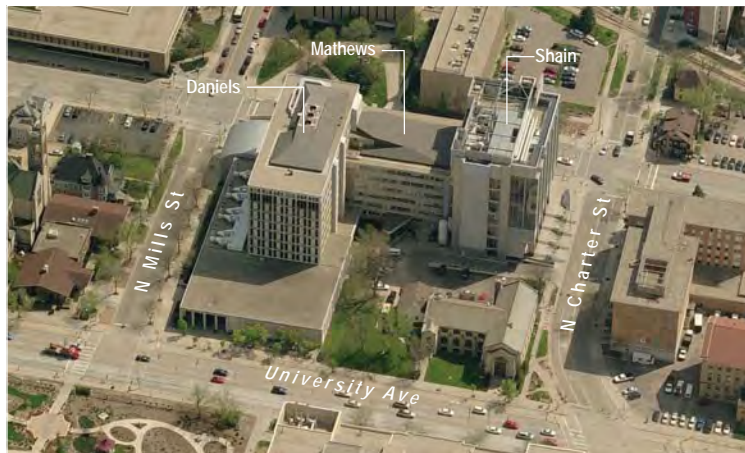
Site Photo from Northwest
