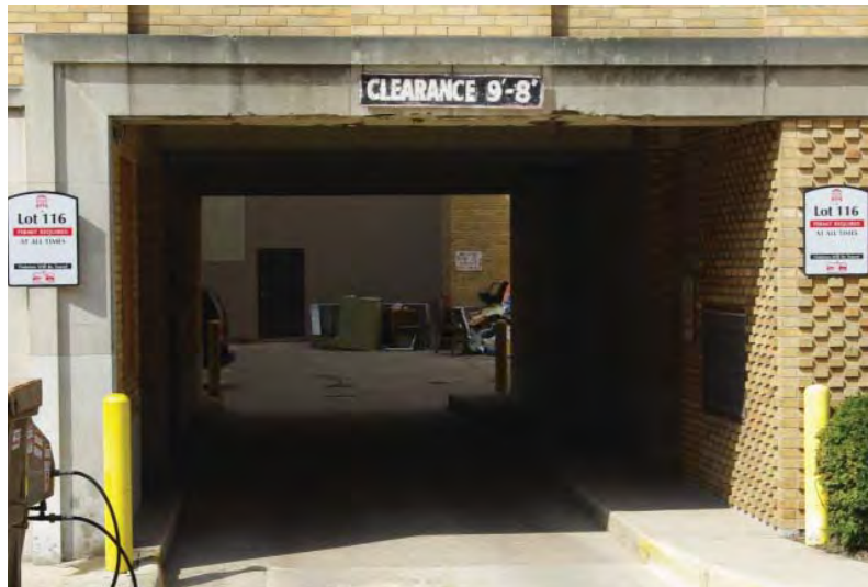
ACCESS TO COURTYARD AND TANK STORAGE AREA
