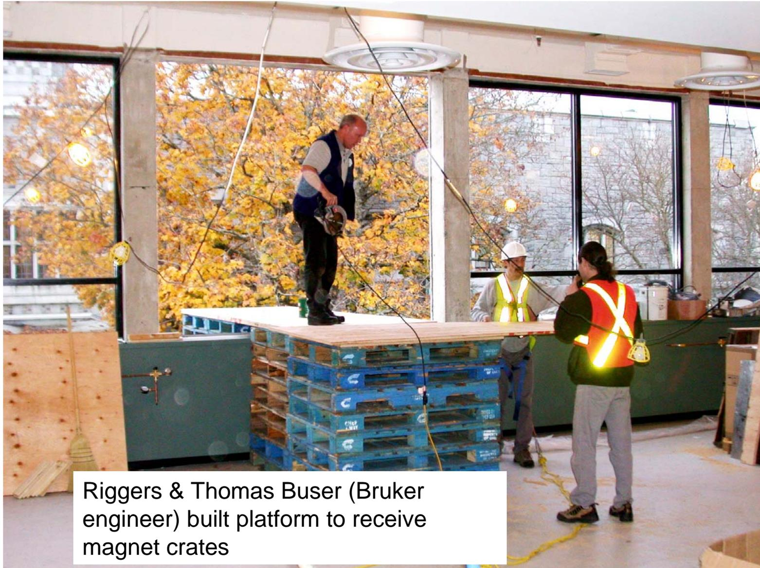
Riggers & Thomas Buser (Bruker engineer) built platform to receive magnet crates
